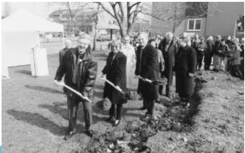
Figure 4 The official start of construction work on the “Hiberniaschule” project, in Herne
