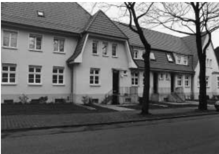
Figure 5 Example of seepage in multi-storey apartment construction
